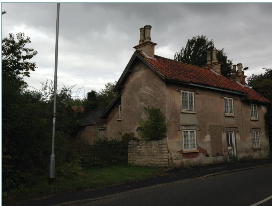
Eddison's Cottage and well-designed former small holding site opposite
